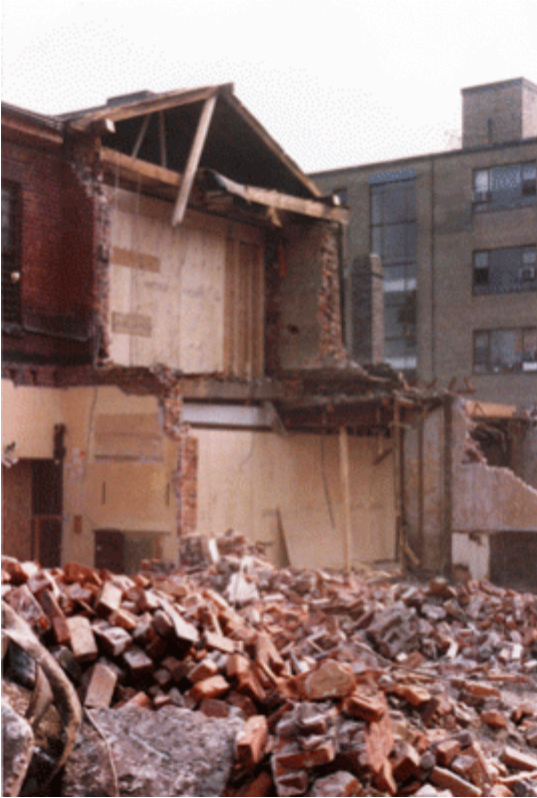
Lambton House about to be demolished (Photo by Madeleine McDowell)
